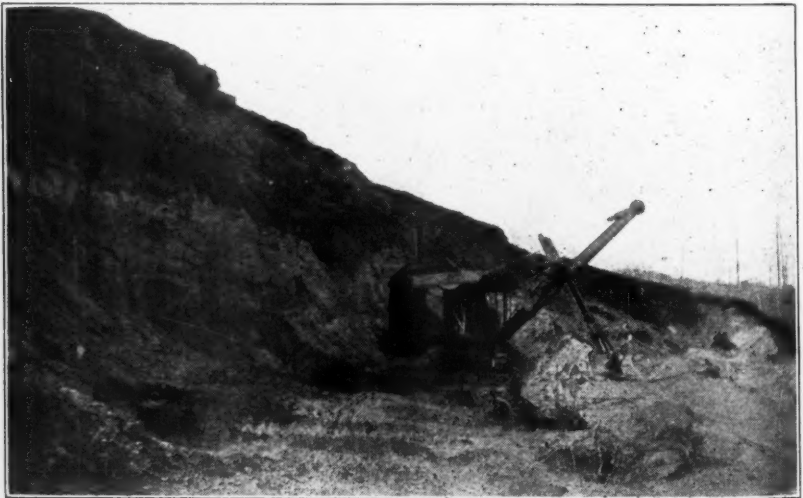
A View of the Pit
